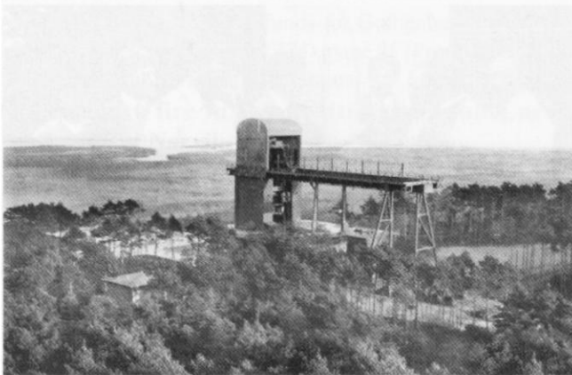
This is test stand number 1, one of several test stands built at Peenemünde. Rockets underwent static tests, and were then launched over the Baltic Sea seen in background
